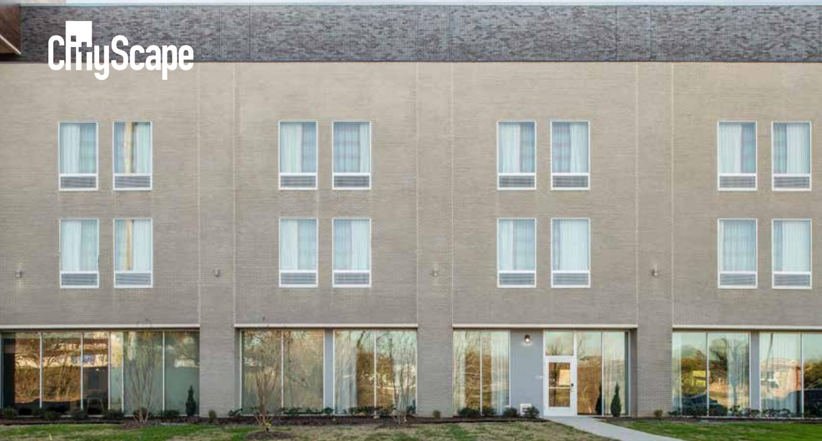
CityScape thinBRiK™ are extruded units, with the added benefit of dovetail slots on the back. They are compatible with formliner systems, or with lightweight metal panel systems where brick are secured with a thinset system and then finished with traditional mortar.
